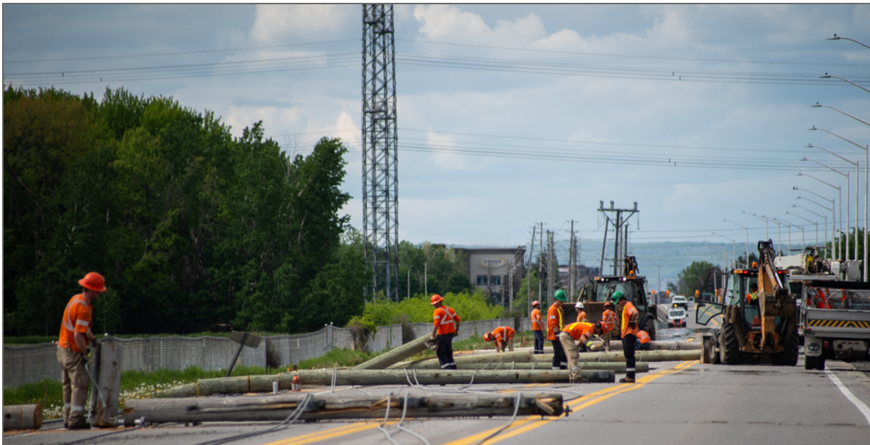
Restoration work after the 2022 Derecho
